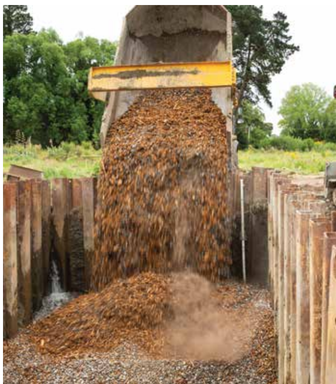
The denitrification wall being installed near Kaiapoi last November 2018.
